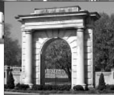
Main Entrance Gate
